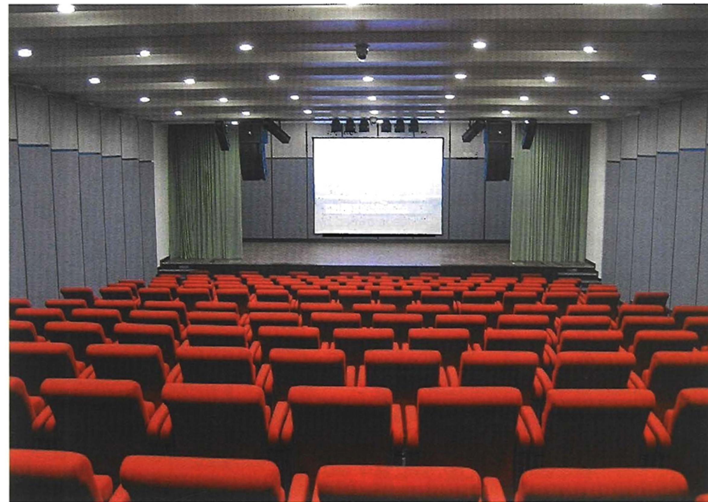
The ADNOC auditorium with JBL VRX line array system
